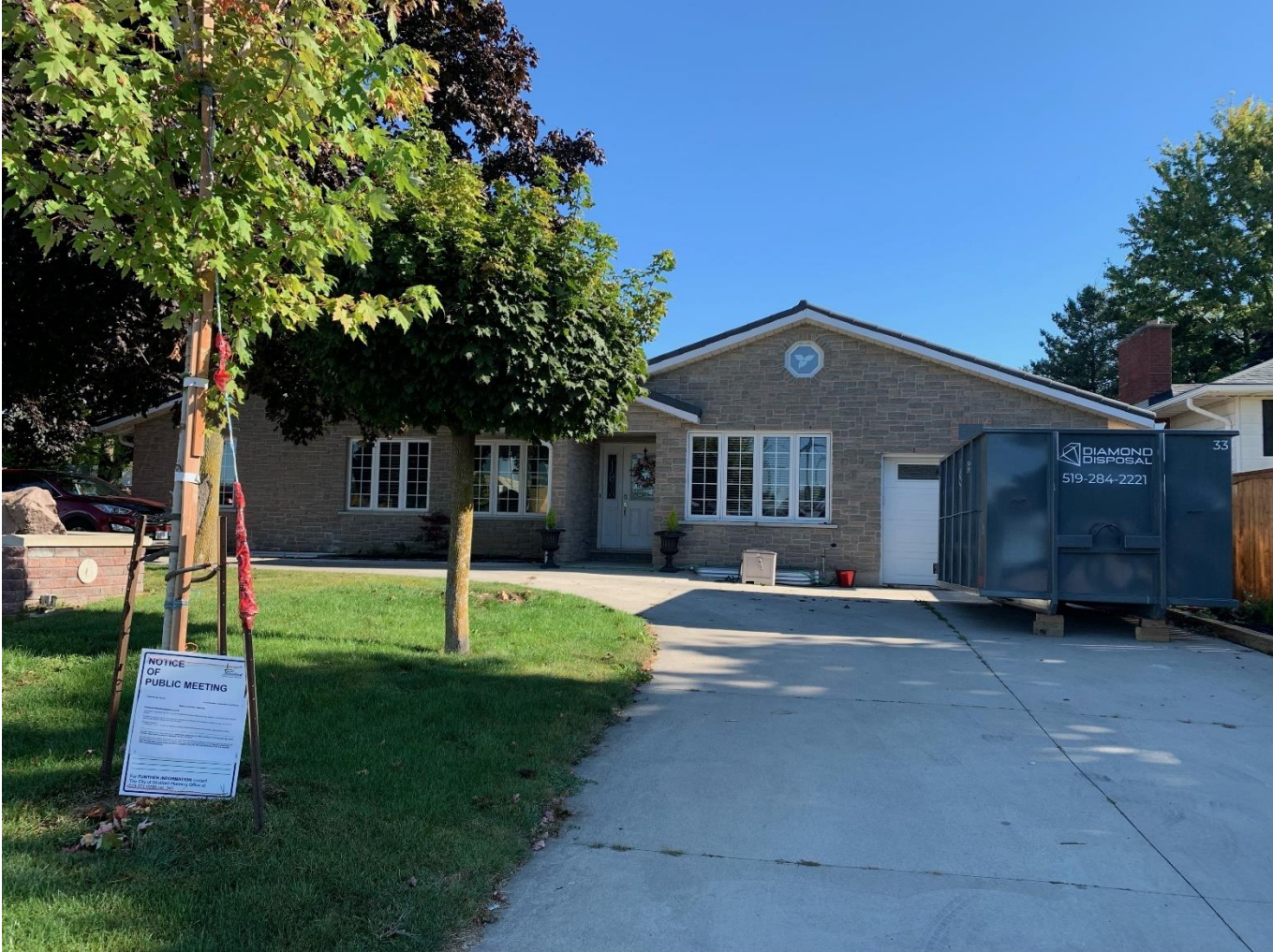
Figure 2 – Site Photo (September 10 th , 2024) File # A24-24 Richard Paradis – 460 Huron Street
