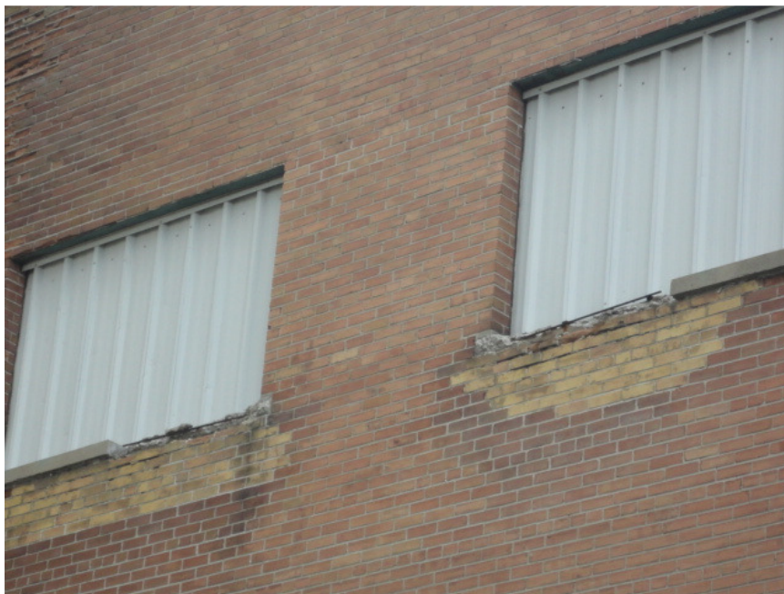
Photo #47: Typical repaired masonry below window sills
