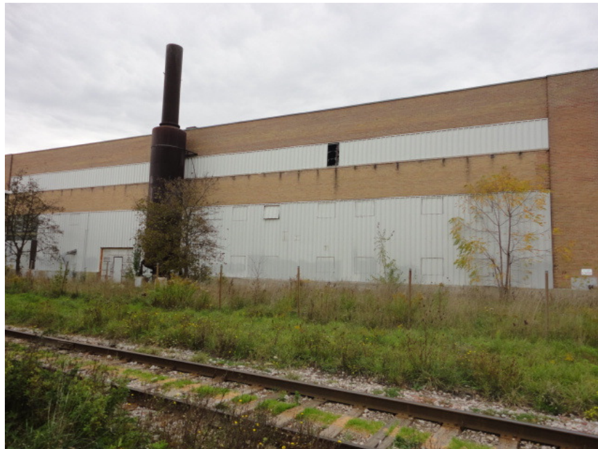
Photo #11: Metal cladding infill of window openings at Addition Bay
