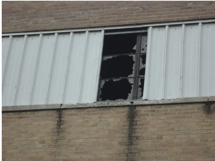
Photo #12: Typical pre-cast concrete window sill
