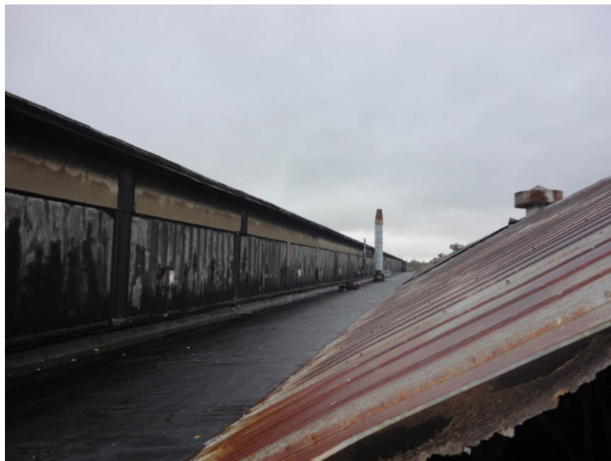
Photo #49: Typical roof assembly and condition
