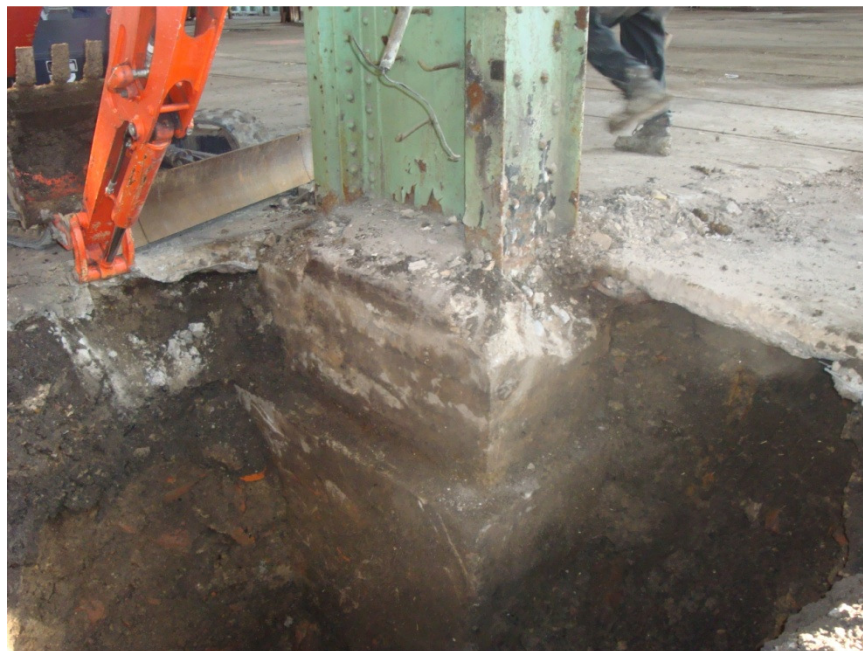
Photo #5: Concrete pier in test pit location
