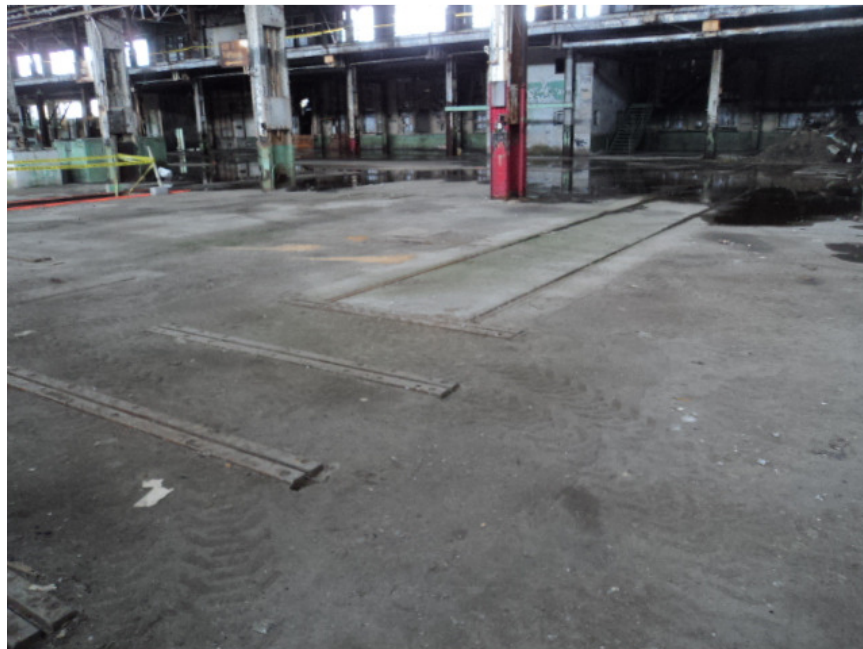
Photo #7: Typical embedded items in slab-on-grade
