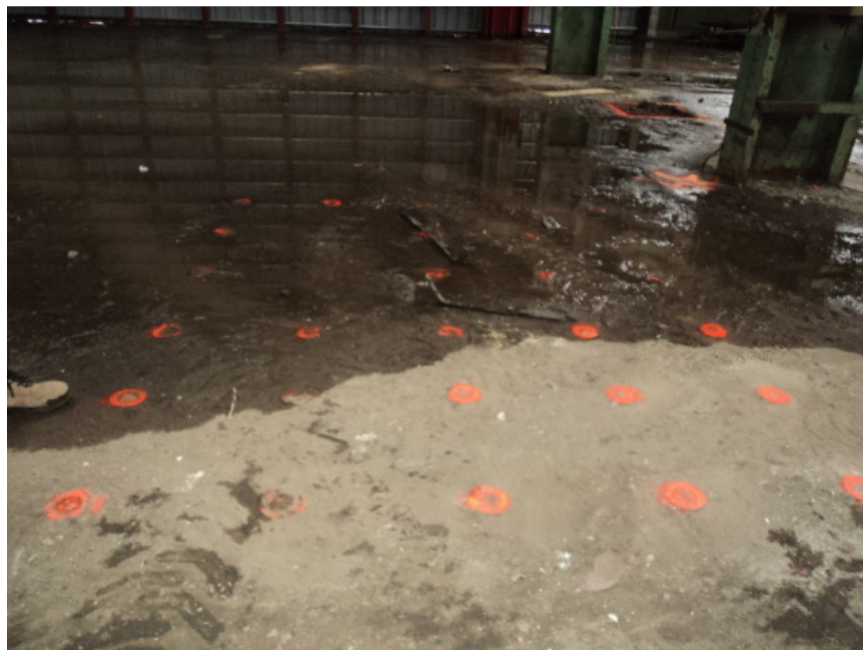
Photo #41: Typical slab-on-grade embedded anchors
