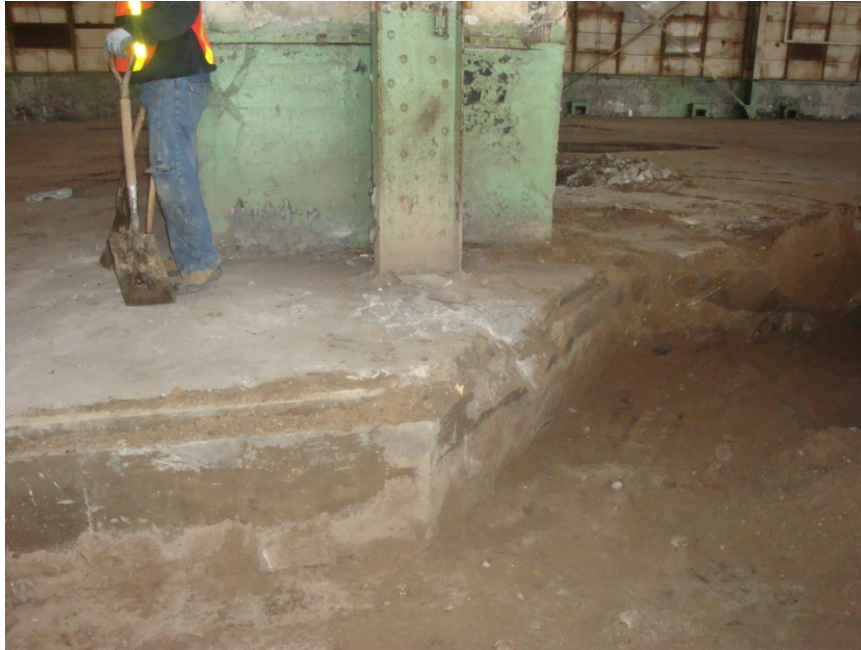
Photo #38: Test Pit #4 - Concrete Pit interference
