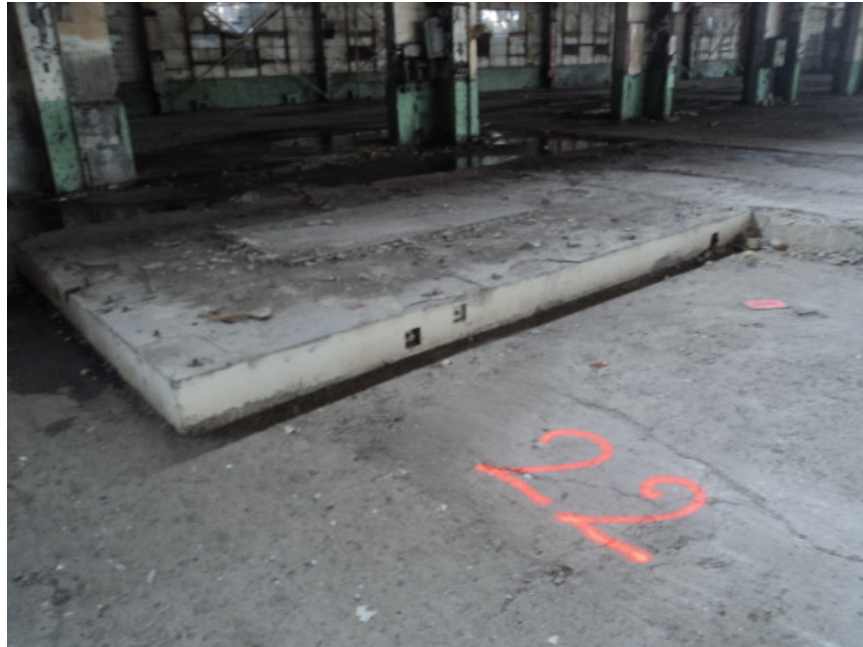
Photo #40: Typical slab-on-grade raised concrete pad
