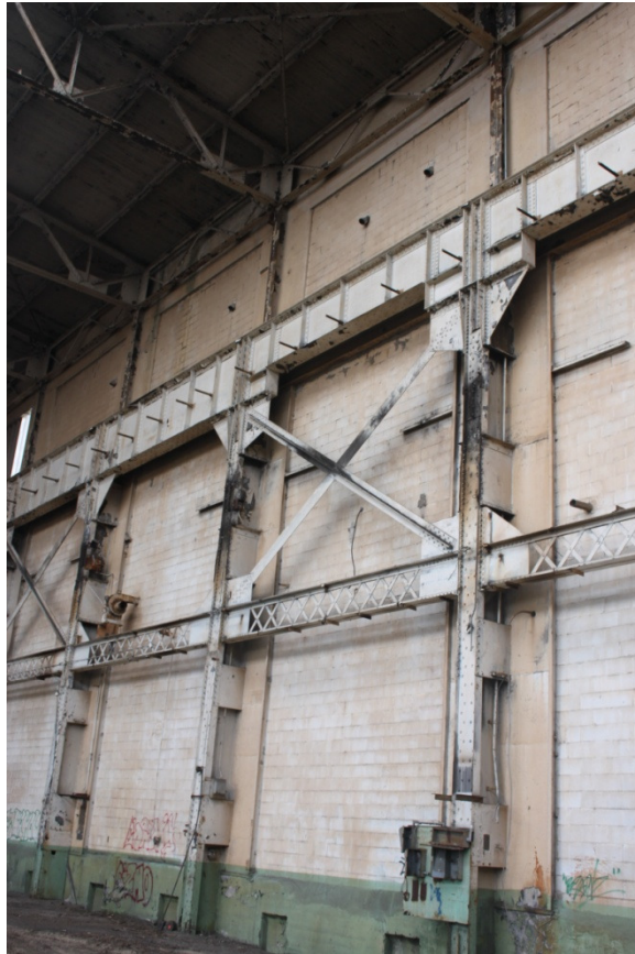
Photo #8: Typical cast-in-place concrete walls with block infilled openings
