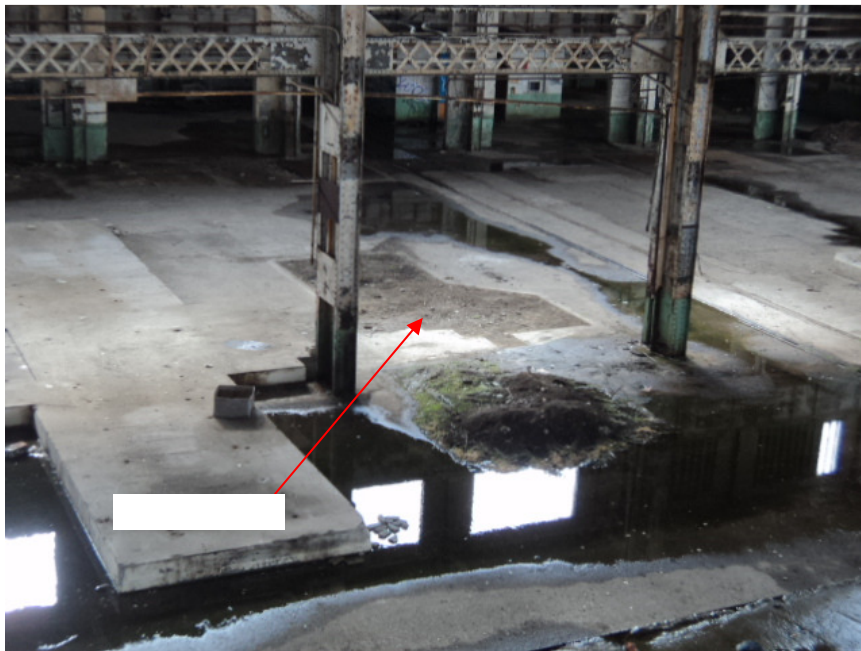
Photo #39: Typical slab-on-grade dirt infill area
