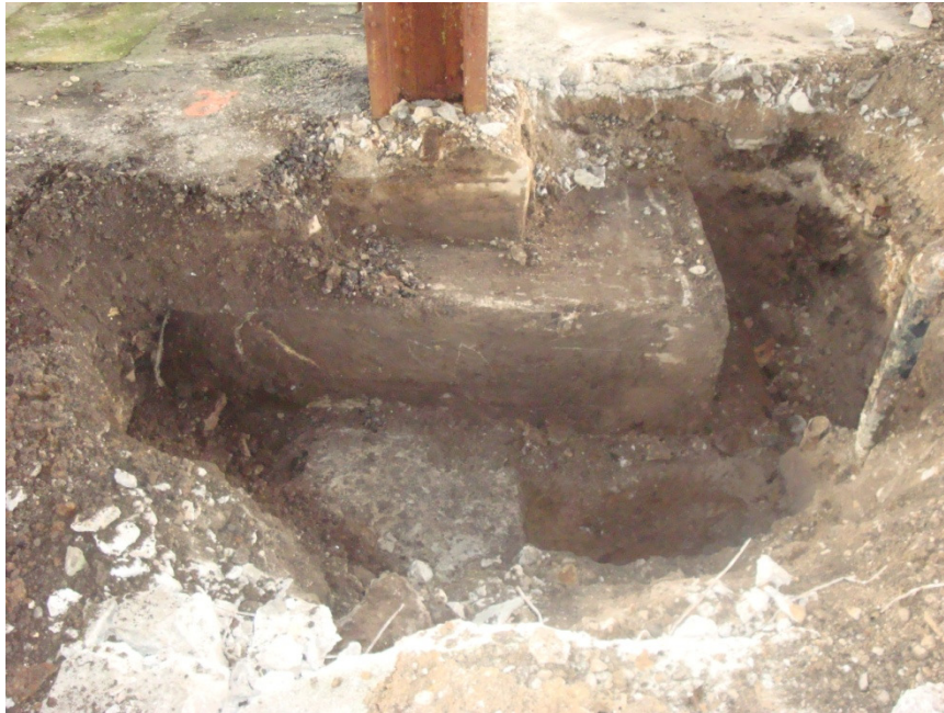
Photo #34: Test Pit #1 - Footing / Caisson Cap
