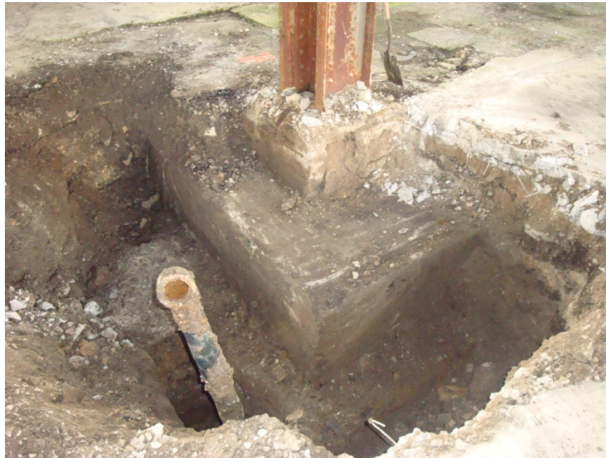
Photo #6: Concrete pier in test pit location
