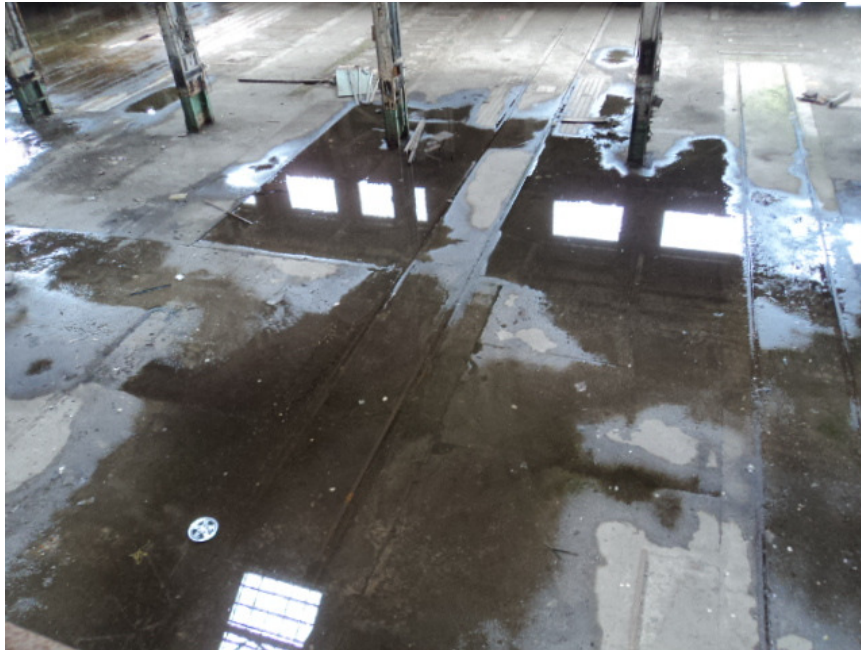
Photo #42: Typical slab-on-grade embedded train rails
