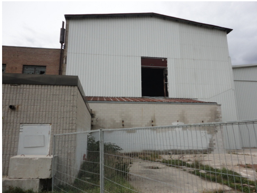
Photo #9: Metal clad segment of the building (west end)
