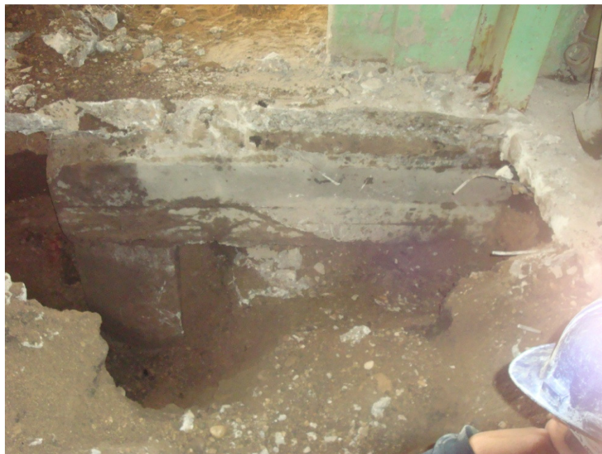
Photo #37: Test Pit #3 - Grade Beam and Piers
