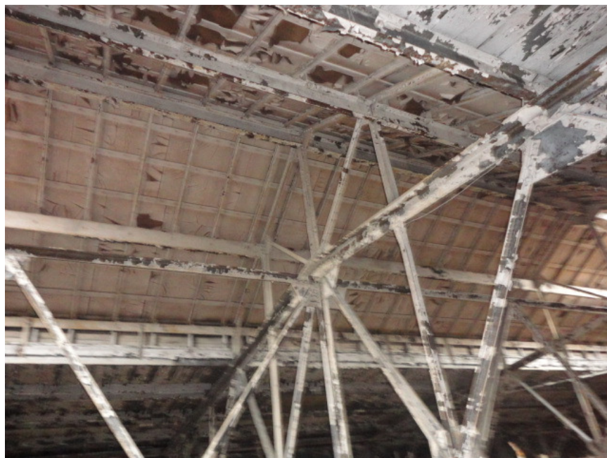
Photo #13: General view of typical roof soffit
