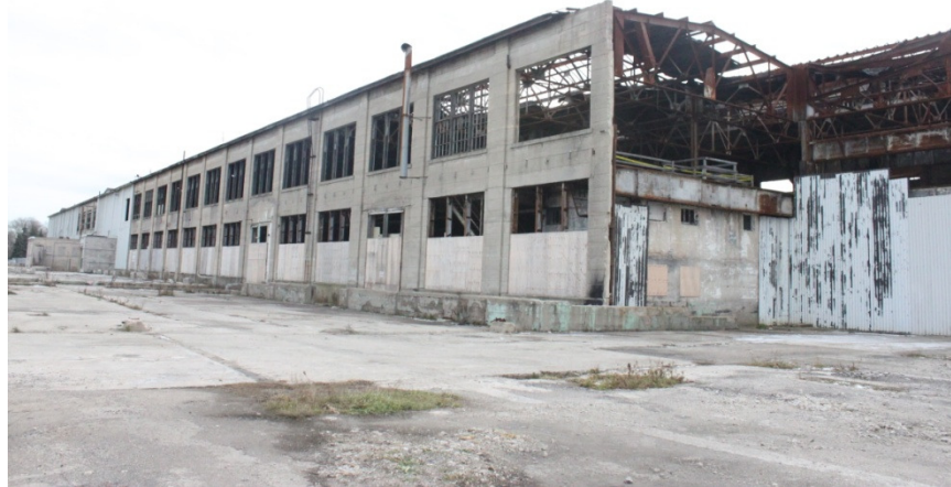
Photo #1: General view of existing building from exterior
