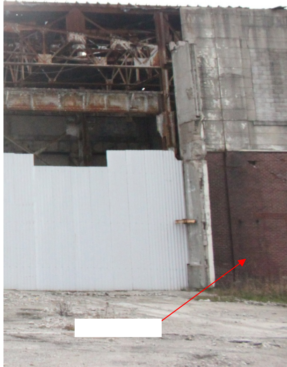
Photo #10: Brick cladding up to mid-height of building (northeast corner)
