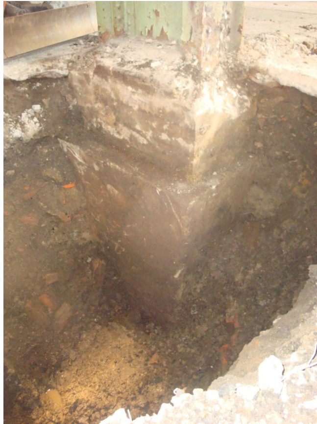
Photo #36: Test Pit #2 - Footing / Caisson Cap
