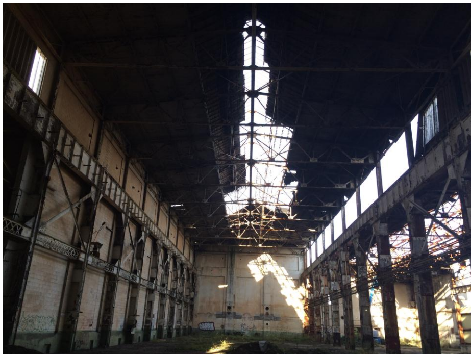
Photo #2: General Overview of the Roof
